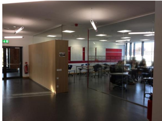
Figure II.0.8 Glass partition between circulation area and classroom
