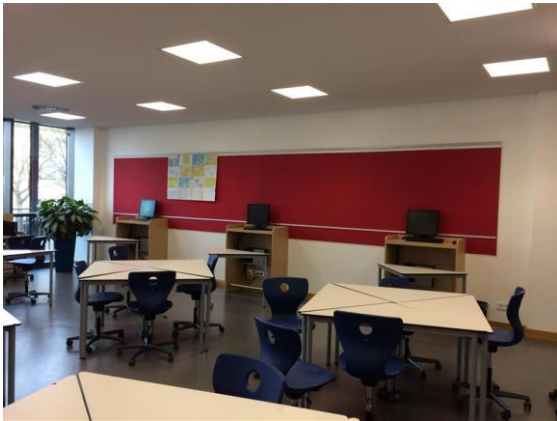
Figure II.0.9 Sound absorbing wallpanels in the break out space
