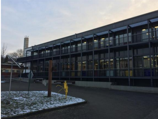
Figure II.0.1 Façade of the renovated building
