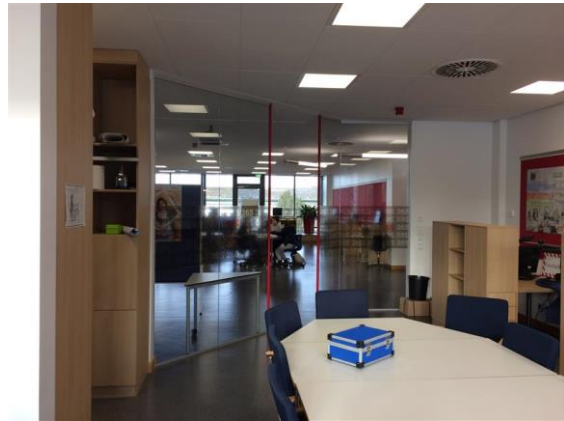
Figure II.0.10 Glass partition between circulation area and teachers room
