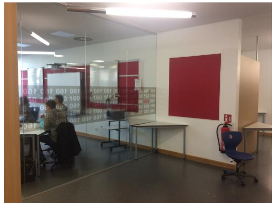
Figure II.0.12 Sound absorbing wallpanel on the side of the circulation area
