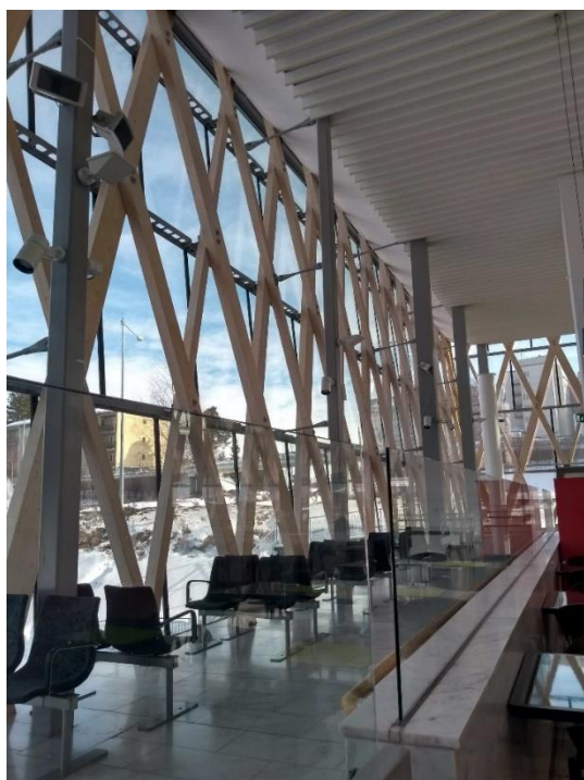
Fig. 5. Umeå bus station. The leaning wall directs sound upwards, the wood crosses diffuse (break) the sound and the ceiling absorbs sound. Photo: John Näsling.
