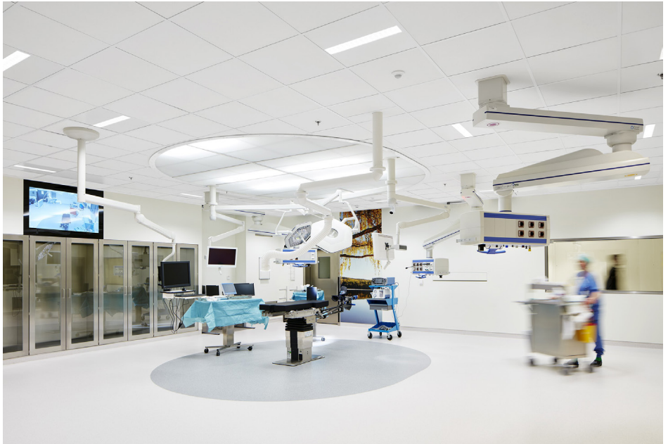
Hybrid operating room 10, 105 m 2
