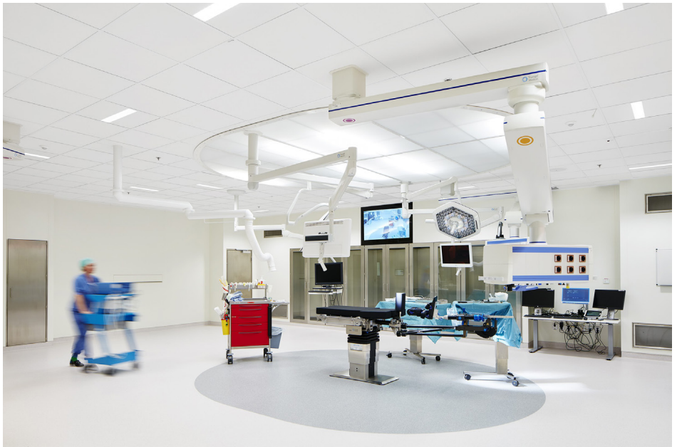
Hybrid operating room 10, 105 m 2
